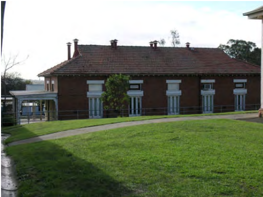
Photograph 22: South west elevation of B6 Source: HLCD, 22.05.07
