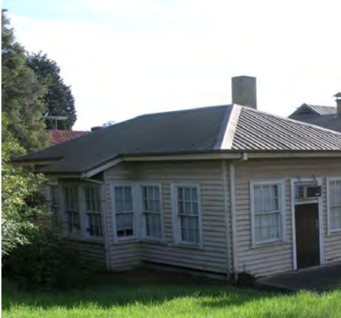
Photograph 13: South west elevation of B3 Source: HLCD, 22.05.07
