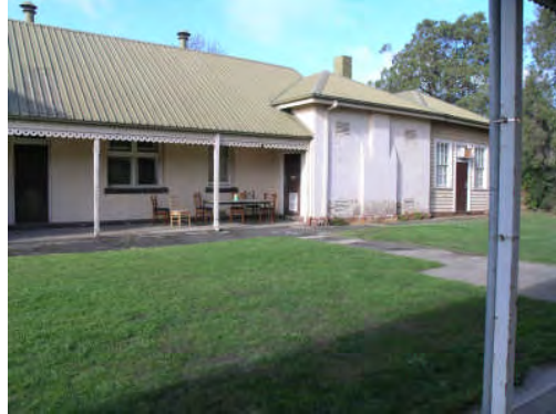
Photograph 14 & 15: North west elevation showing removed chimney stack and later vents on either side of chimney Source: HLCD, 22.05.07
