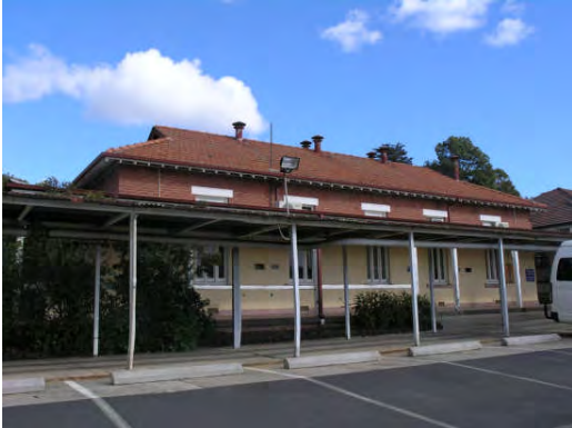
Photograph 21: North east elevation of B6 Source: HLCD, 22.05.07
