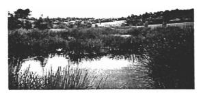
A constructed wetland system is a shallow waterbody system designed to regularly fill and drain. Wetlands tend to be heavily vegetated with emergent aquatic macrophytes which facilitate the removal of fine particulates and soluble pollutants. Wetlands are generally comprised of:
