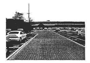
Porous pavements are an alternative to conventional road pavements. They consist of modular pavements cells with gaps between cells to allow infiltration of stormwater.
