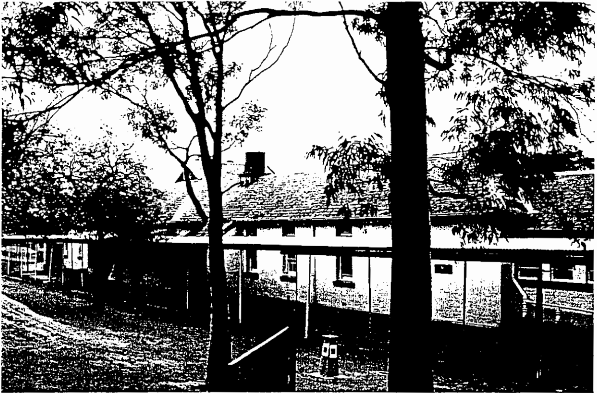
Plate 3: Unit 9 – one of c1889 original buildings
