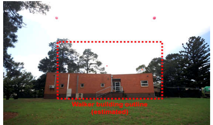
Figure 3 - Annotated view from Main Drive, camera location 1, 1.7m height, 22mm eq. lens
