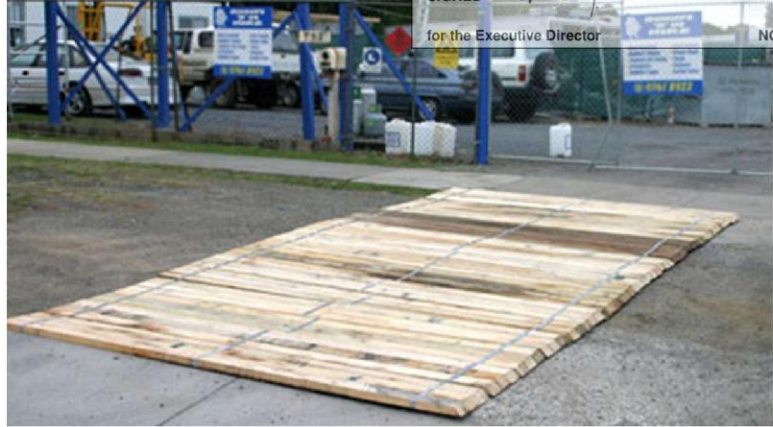
Figure 3: Indicative detail of ground protection - from AS-4970 Protection of Trees on Development Sites. p.17
